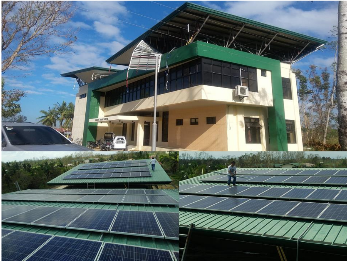
Figure 9. Damaged sidings of the climate change center building and intact/undamaged roof installed with PV panels after Typhoon “Rosita” in October 2018.
