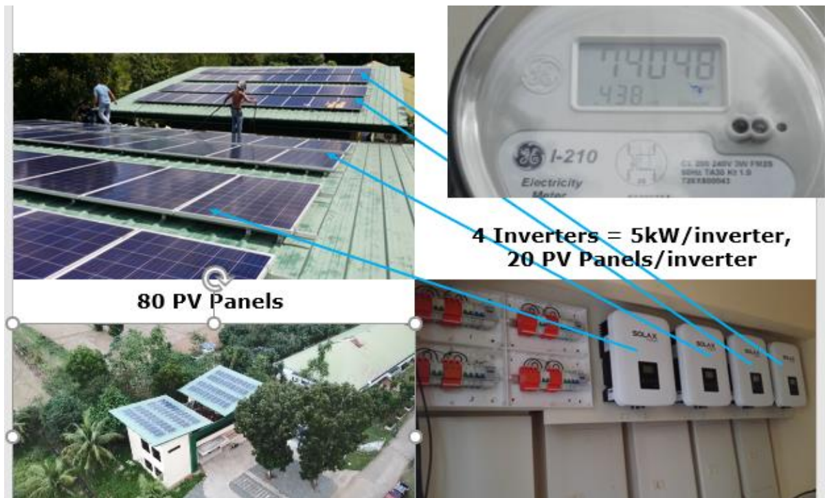
Figure 1. Roof-mounted photovoltaic system of the climate change center building comprising 80 solar/PV panels and four 5-kW inverters connected to the main circuit breaker.
